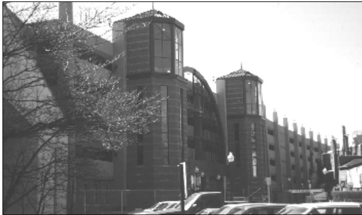
Figure 17. Parking Facility, South Norwalk, CT
