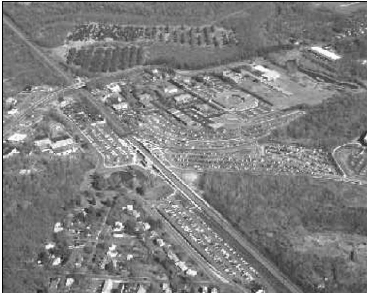
Figure 21. Princeton Junction aerial
